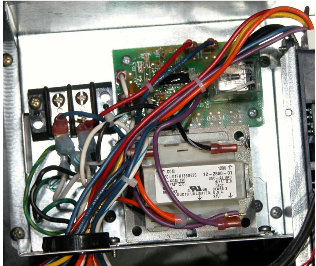
Box purposely mounted at an angle
